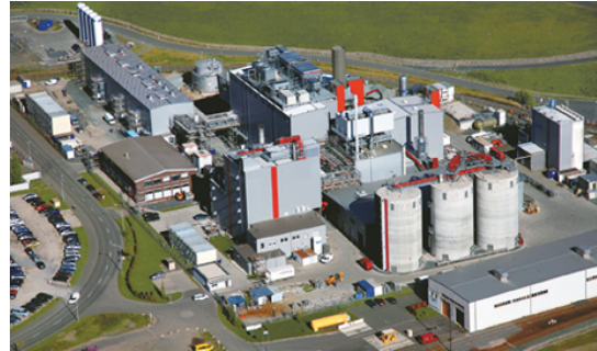
Former CHOREN Biomass Gasification Plant in Freiberg, Germany
